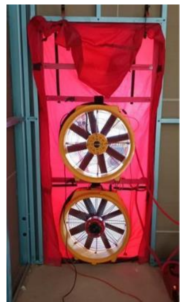
Figure 1. Air permeability testing fans during construction phase of a VHBA project
